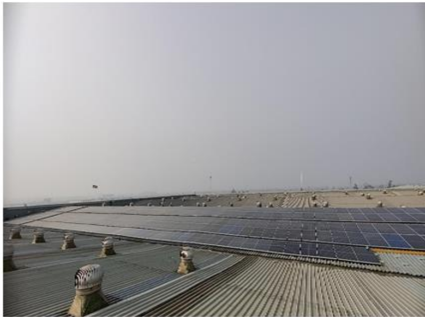
Solar PV Modules Rooftop Installation
